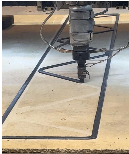
Figure 3: Printing in Progress.
